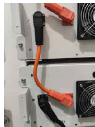
Communication Cable Connection Diagram for Two Battery Packs
