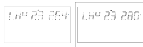
Figure 3-41 Setting the mains High voltage point in inverter mode
